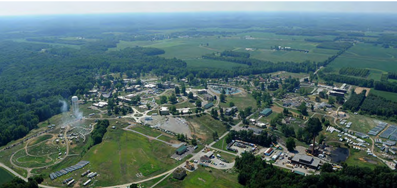
The Muscatatuck Urban Training Center in Jennings County is the largest urban training facility in the country.
